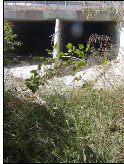
View of site (S) toward Hwy 126
