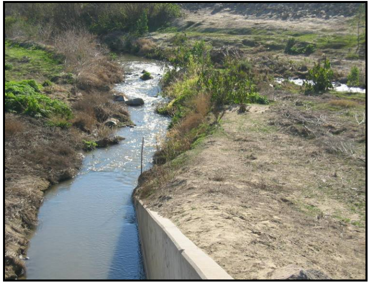
View toward SW looking downstream an ag drain before the confluence with Revolon
