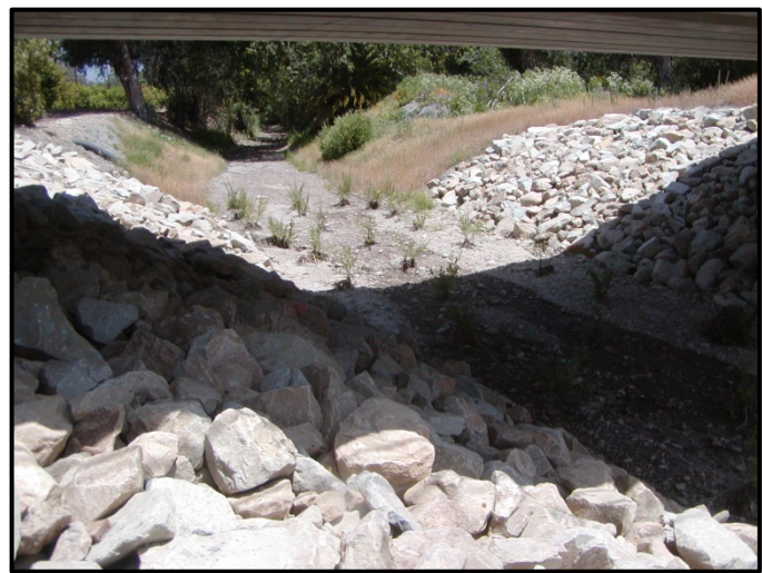
View upstream at the bridge
